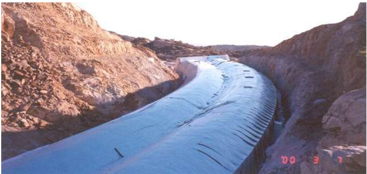
Cut & Cover Tunnel under construction
