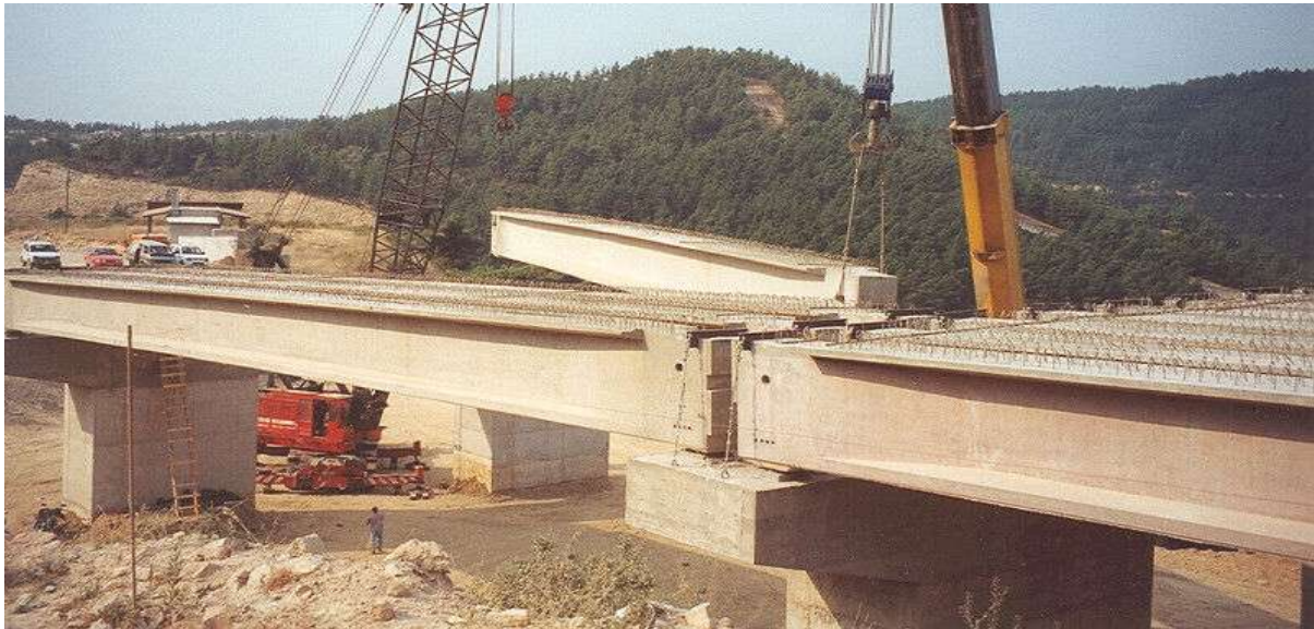
Bridge 103.36m long (34.19+34.98+34.19) at chainage 1+100.0 constructed with precast beams
